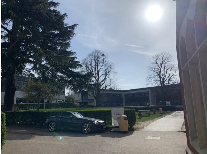
L-block and M-block, as viewed from Gadsden Lawn—2022
